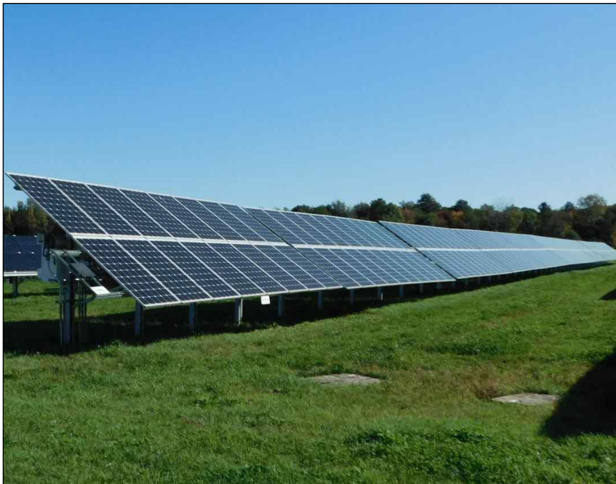
Figure 12 Typical Single Axis Tracking System with Two Modules in Portrait Orientation
