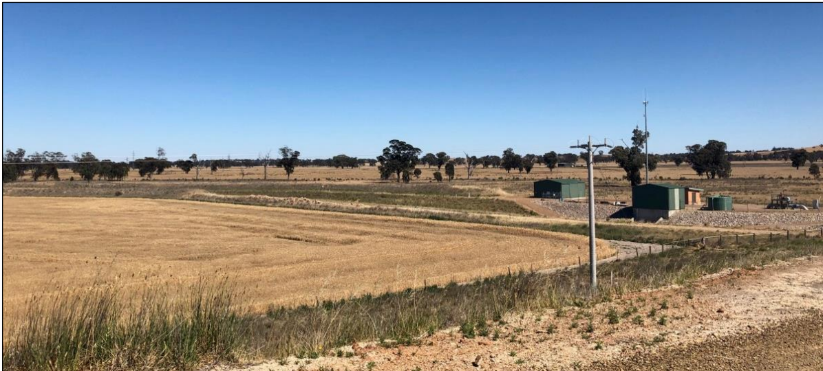
Figure 10 Winton Wetlands Infrastructure (internal drainage basin infrastructure)
