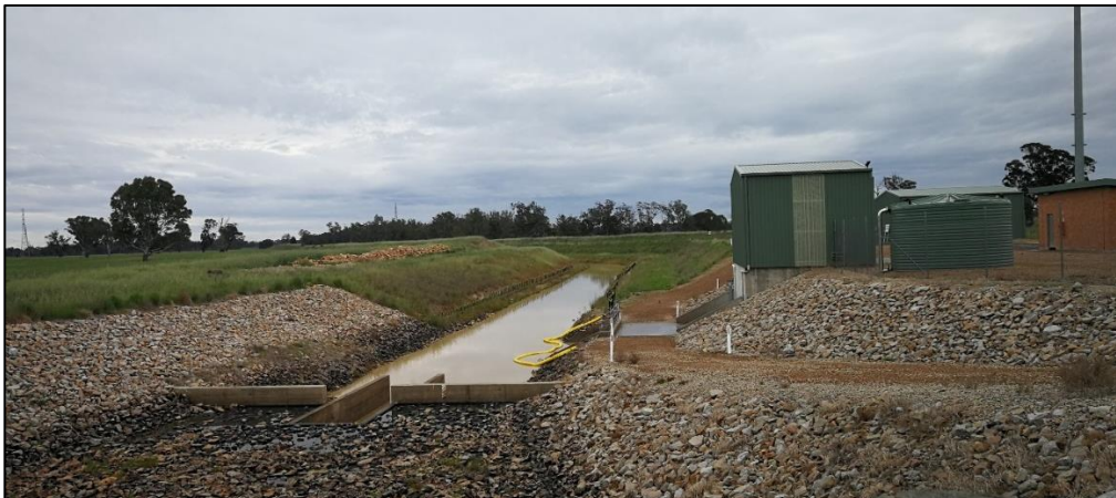
Figure 1 Stockyard Creek Channel looking south from Winton Wetlands
