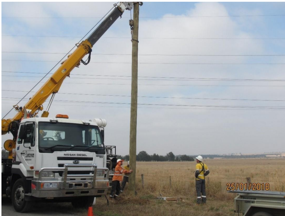
Figure 4. Example of new pole being installed
