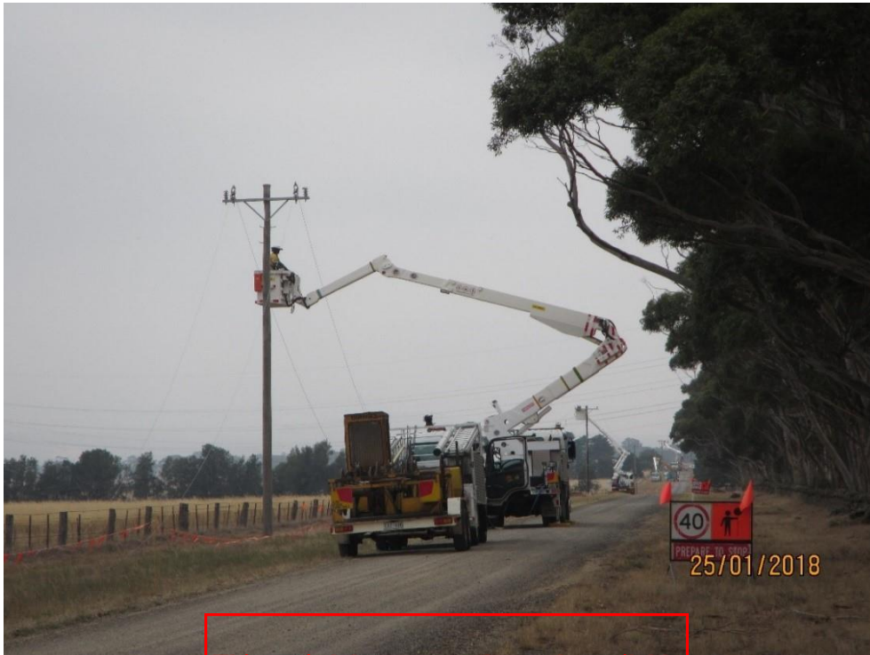
Figure 2. Example of how pole top works are undertaken
