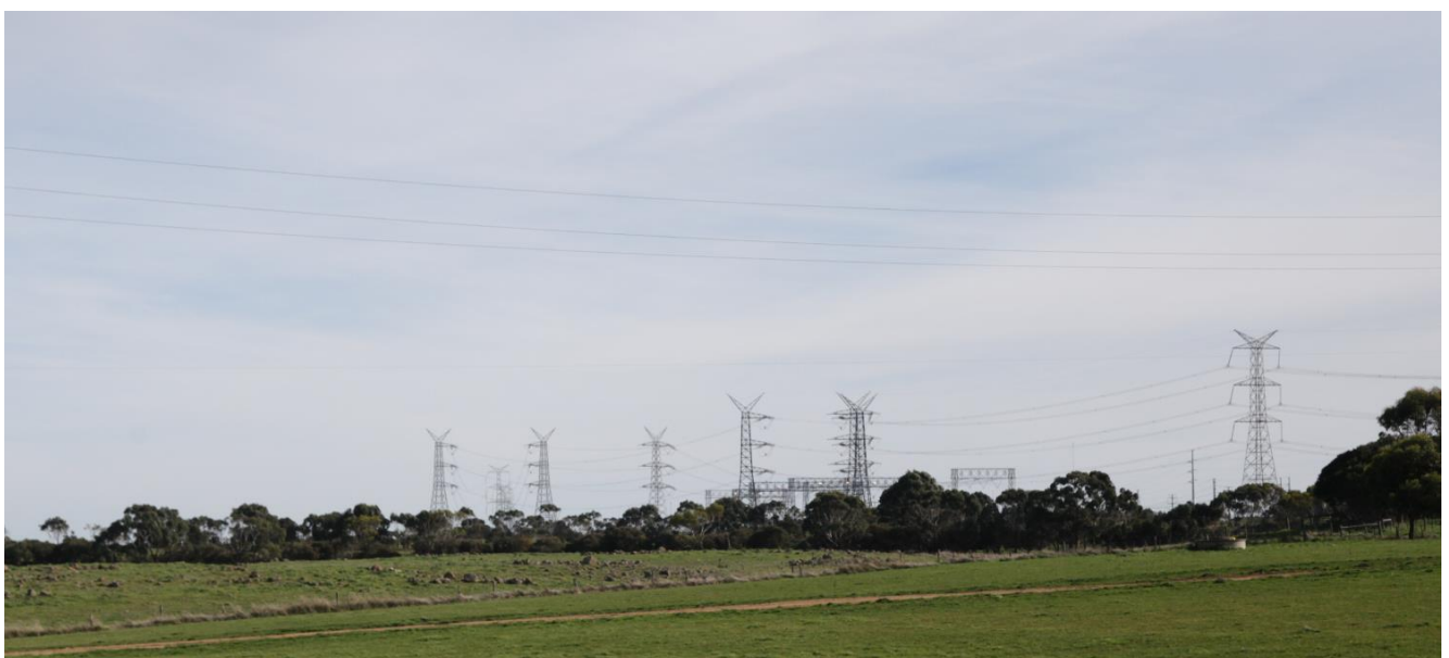
Figure 5-10 Landscape Character Unit 6 – Infrastructure example
