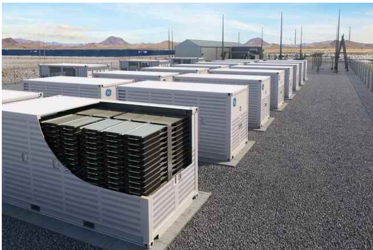
Figure 3-5: Typical BESS Arrangement
