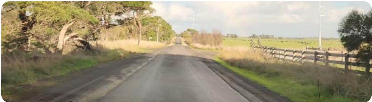
Figure 3 Tarrone North Road facing South towards Riordans Road
