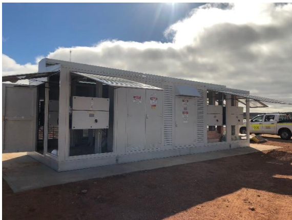
Above is an example of Skid mount inverter/transformer station
