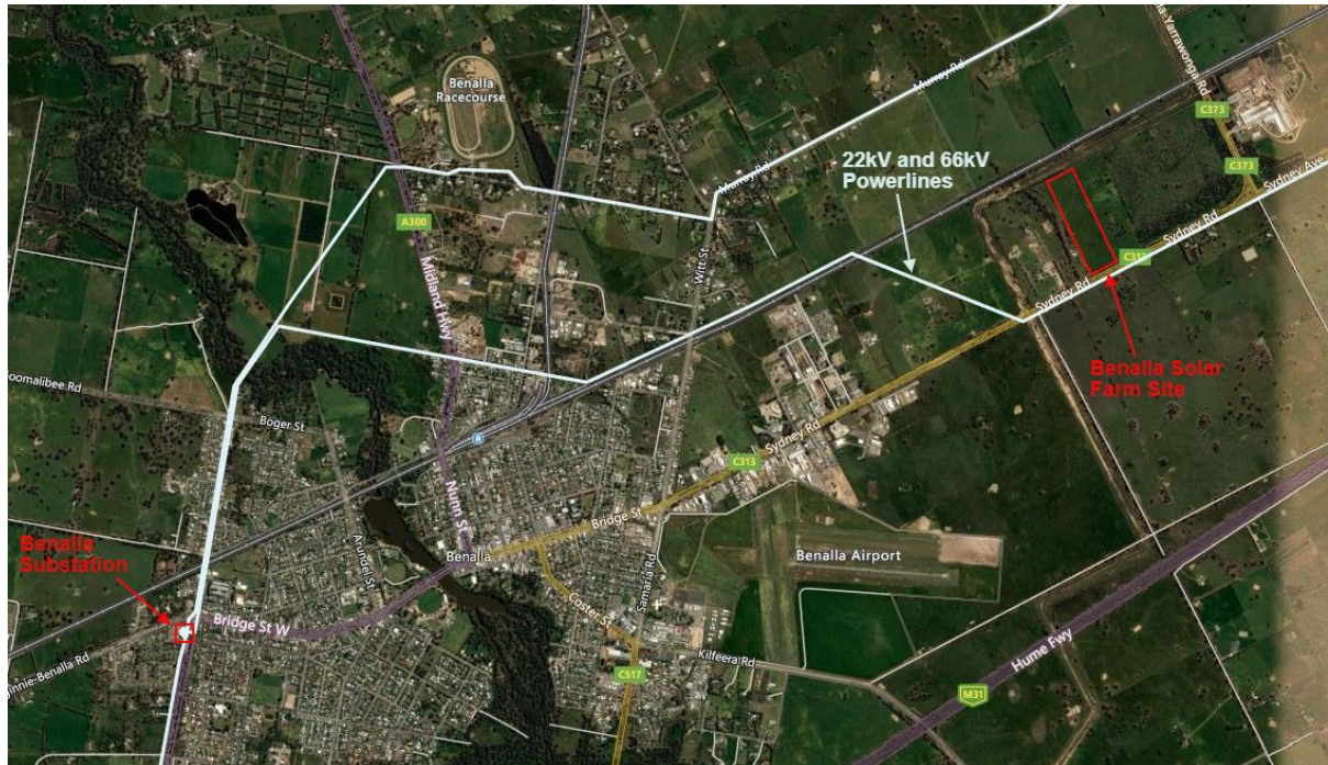
Figure 1 – Benalla Solar Farm site showing Benalla substation and the 22kV and 66kV feeders
