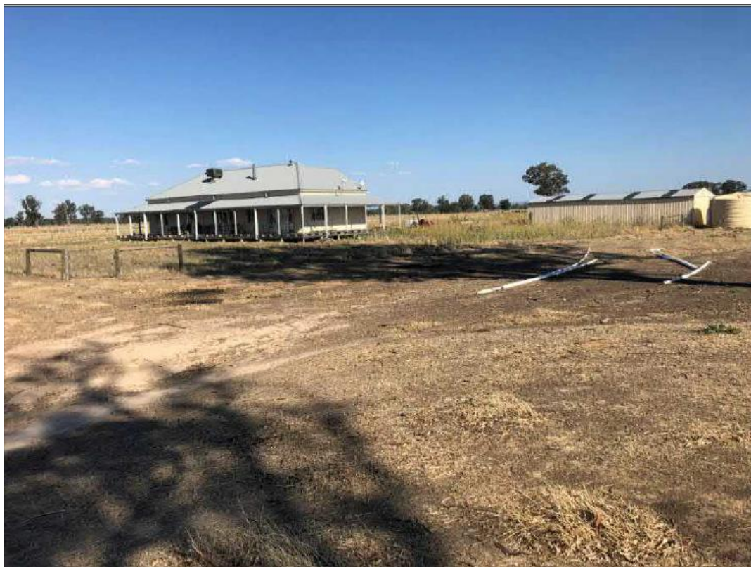
Figure 4 Dwelling and associated outbuildings at 51 Nelson Road, looking north west.
