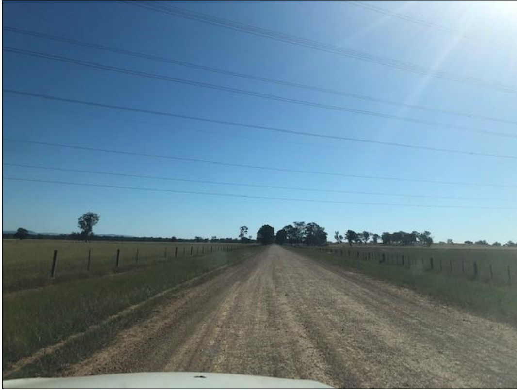
Figure 5 Unsealed Nelson Road running along the southern boundary of the site
