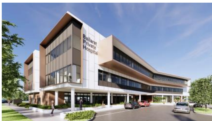
EXTERNAL VIEW - SOUTH EAST CORNER
