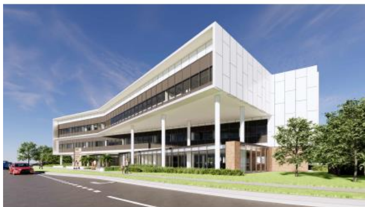
EXTERNAL VIEW - SOUTH WEST CORNER
