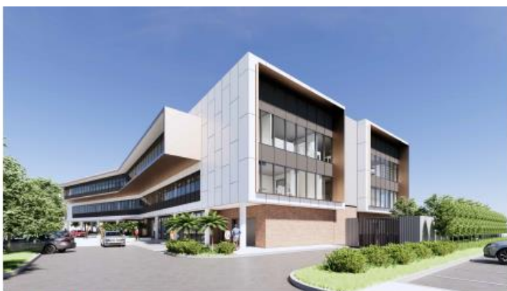
EXTERNAL VIEW - NORTH EAST CORNER
