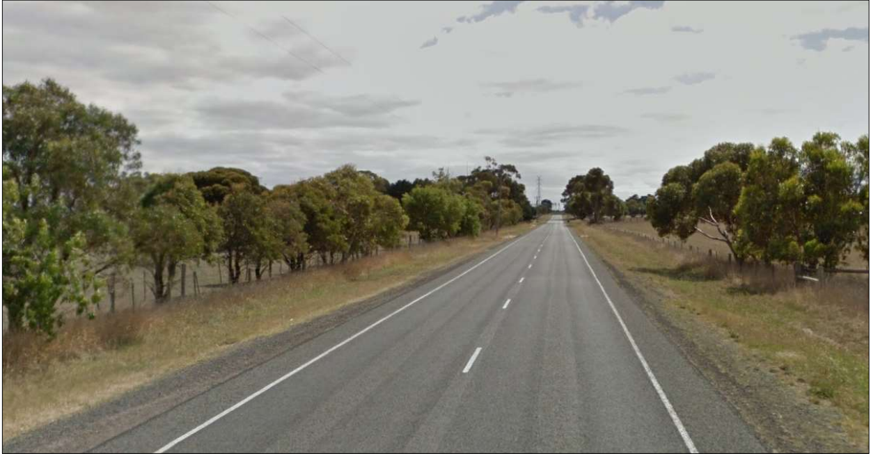
Figure 2-5: View of Ballan Road (Source: Google Street View, 2020)
