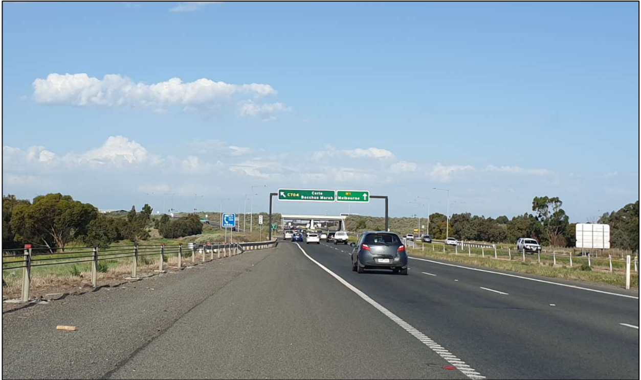
Figure 2-2: View of Geelong Ring Road
