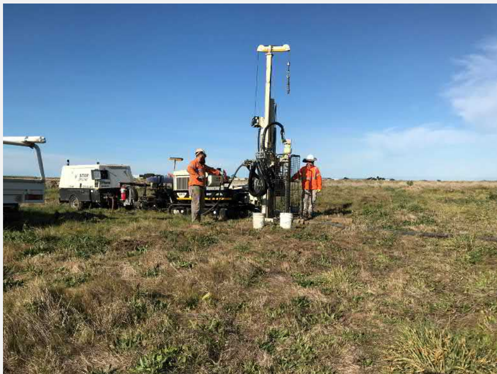
Plate 15: Groundwater well installation at MW001
