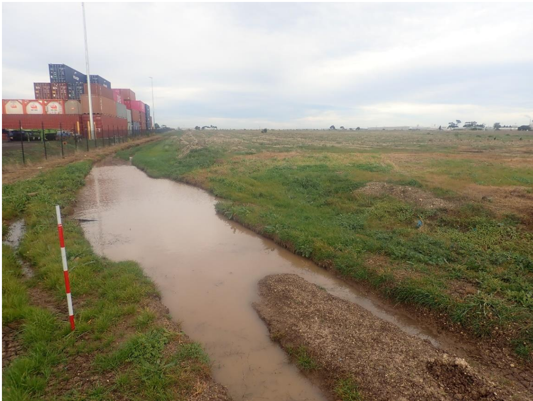
Figure 11 Lying water over exposed clay soils within eastern extent of Project area (B. Watson 7/05/2020)
