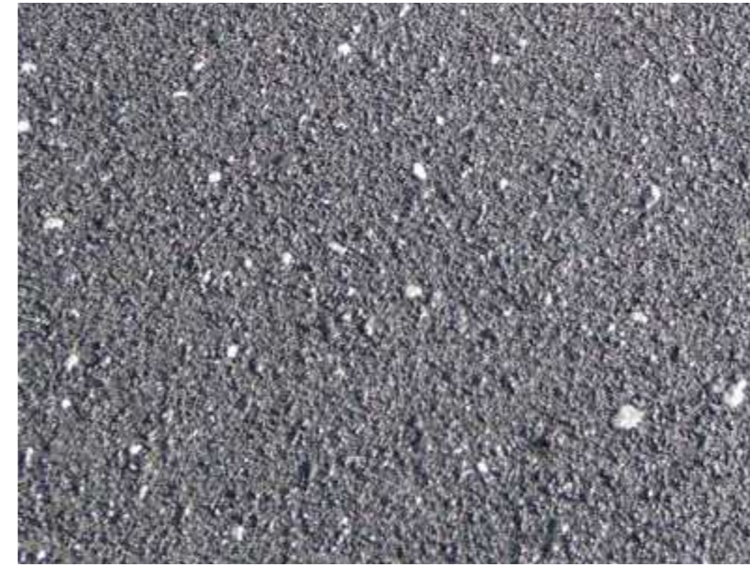
Concrete hardstand to engineers specification)
