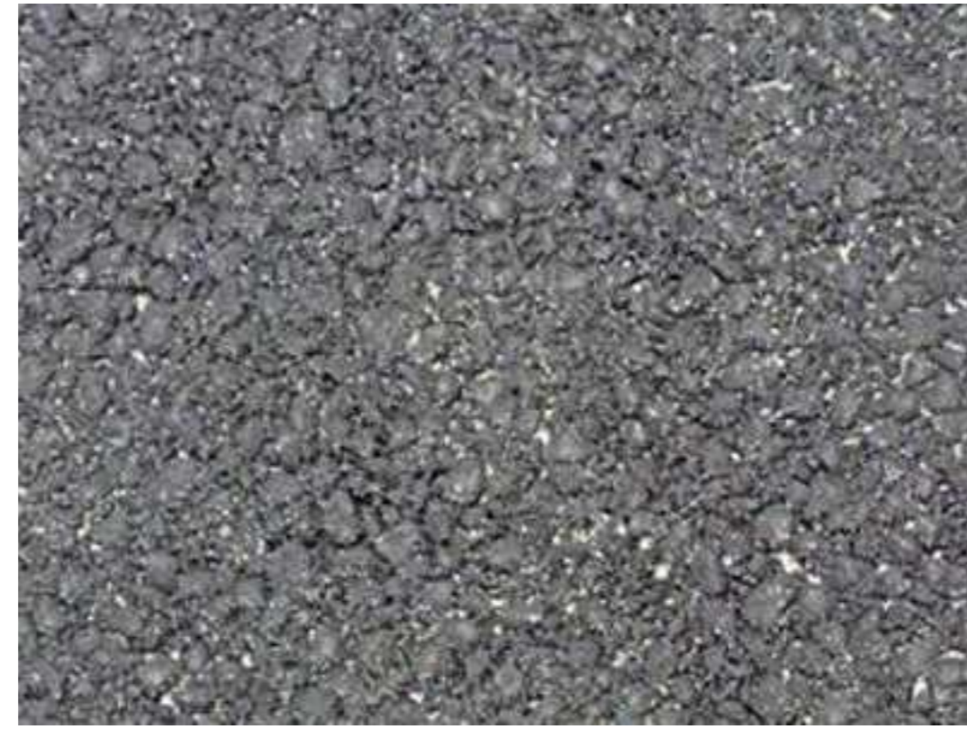
Bitumen hardstand to engineers specification
