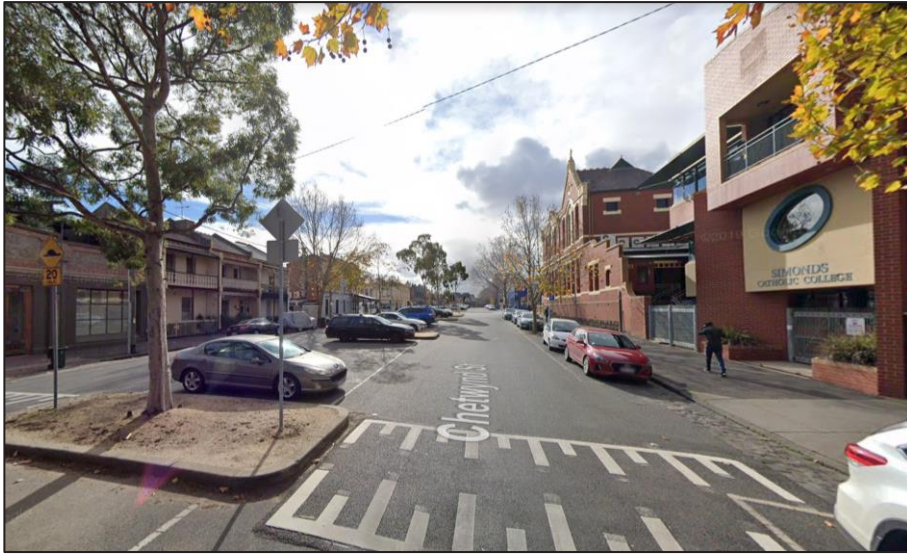
Figure 2.4: Chetwynd Street looking north adjacent to the Subject Site
