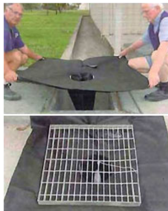
Figure 5.3: Drain Warden (Reference: Melbourne Water)
