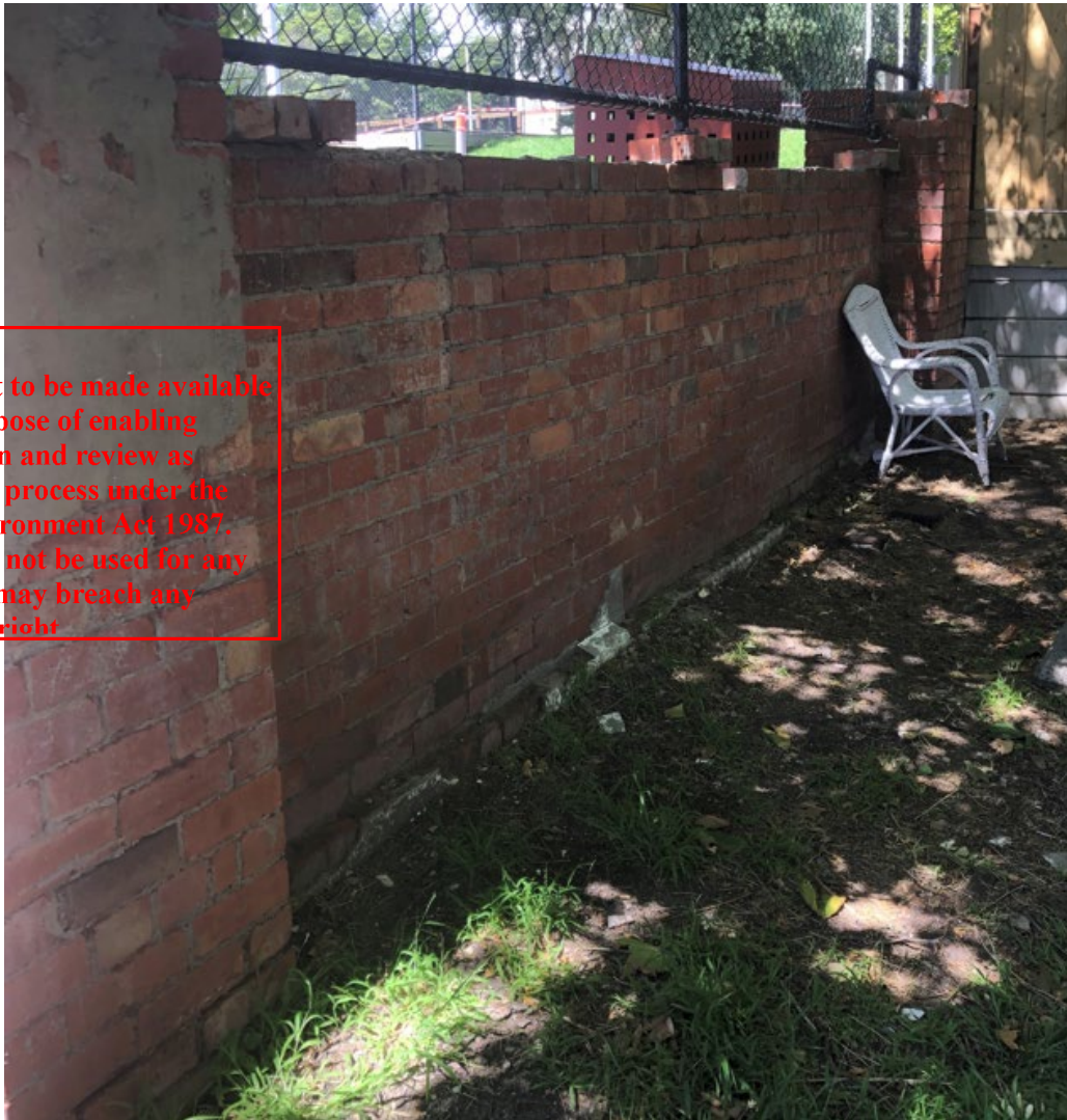
Figure 10. View of existing masonry fence. (Justin Herbert, 3 December 2021).
