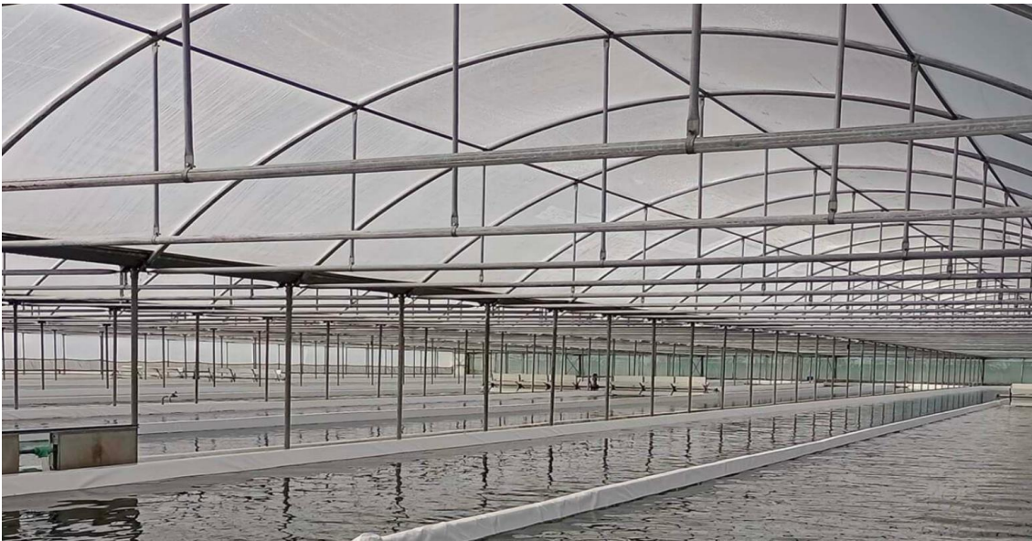
Example of raceway ponds and greenhouse structure proposed for micro-algae cultivation (Source: C-Loop)
