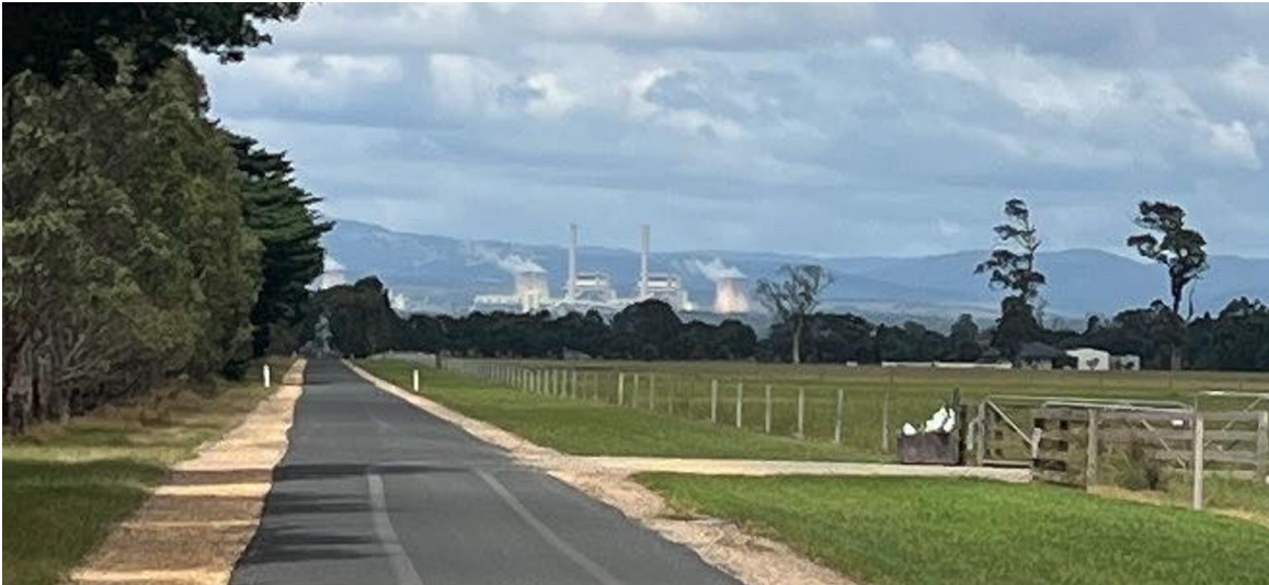
Loy Yang Power Station from River Road (Date of photograph: 26 January 2024)
