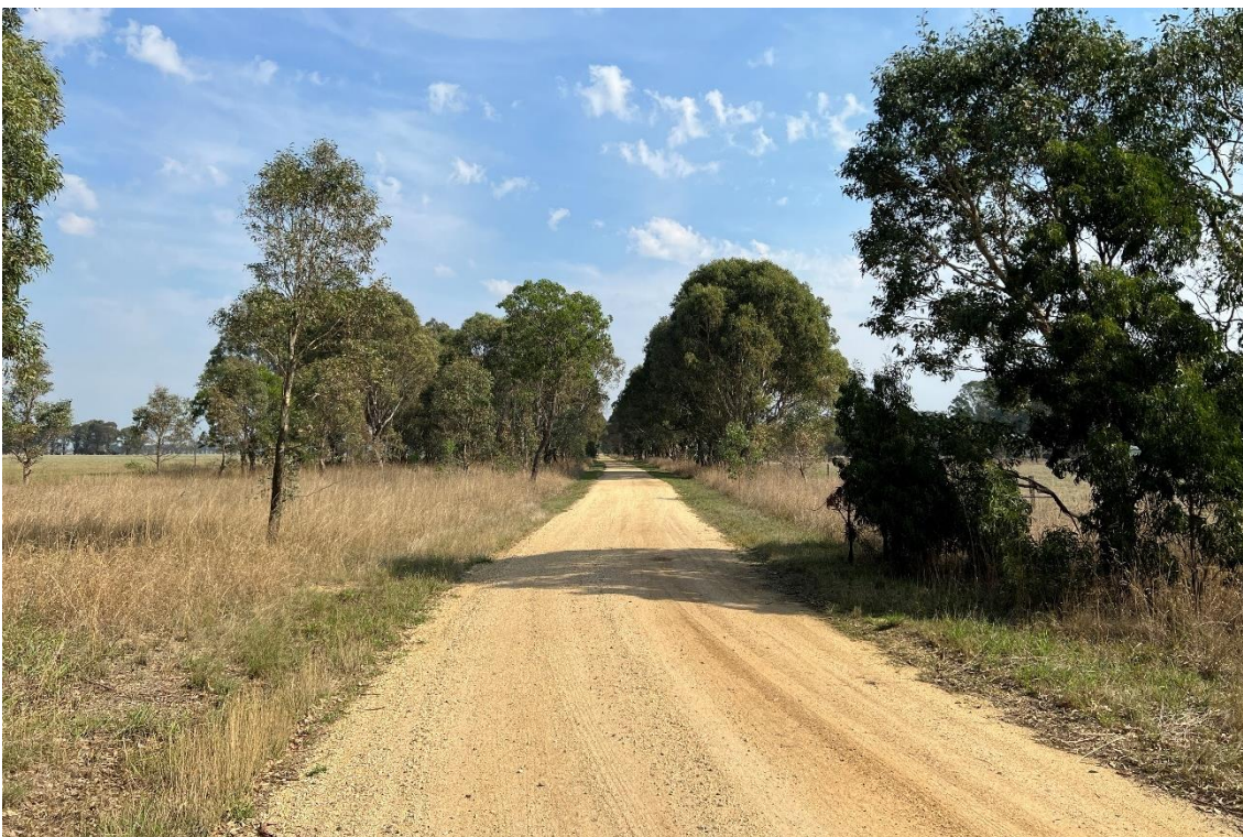
Looking west along Hendersons Road from intersection with Graham Road (Date of photo: 7 April 2023)
