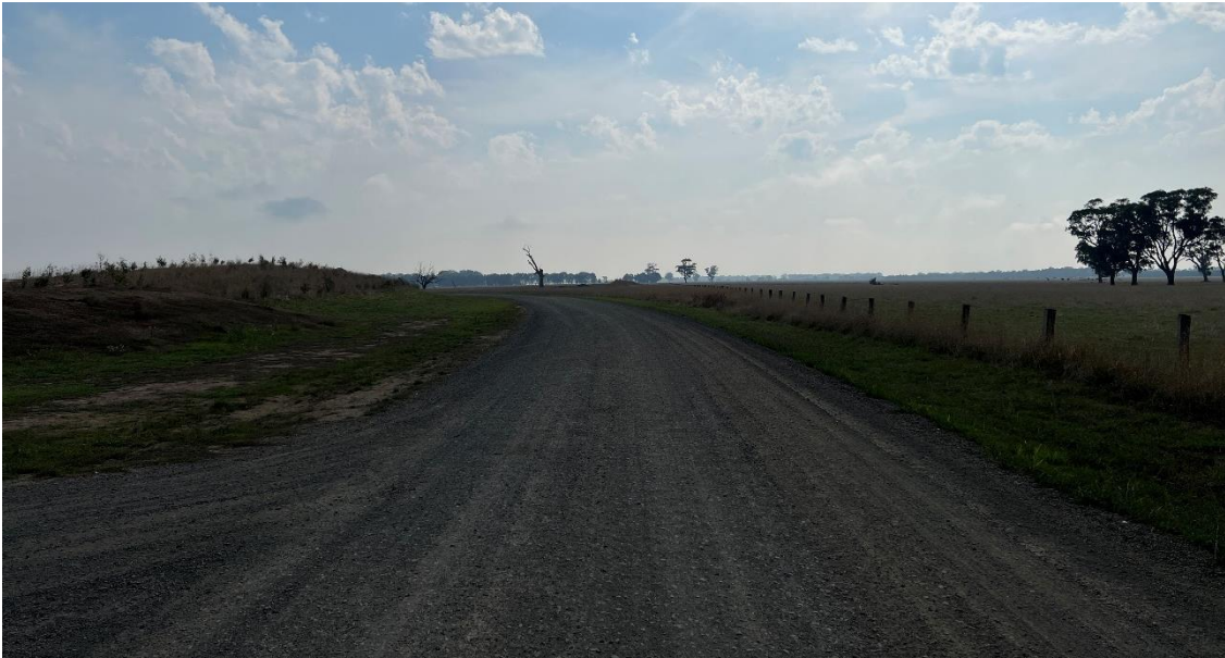
Looking north along existing accessway curving to the north-east from Graham Road (Date of photograph: 7 April 2023)
