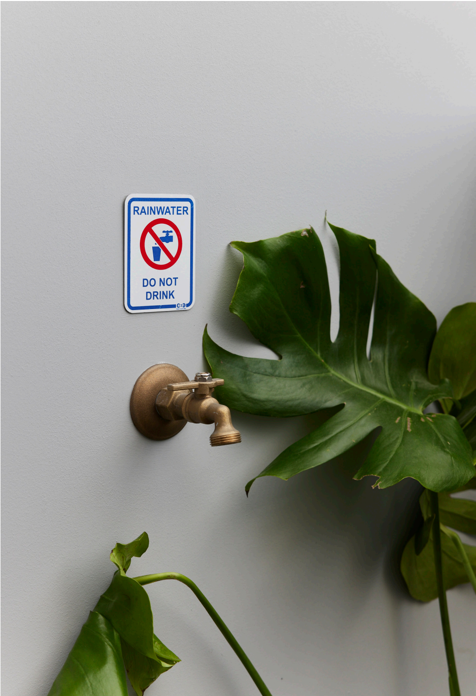
Rainwater connections to balcony taps at Ferrars & York. Photography by Kim Landy.
