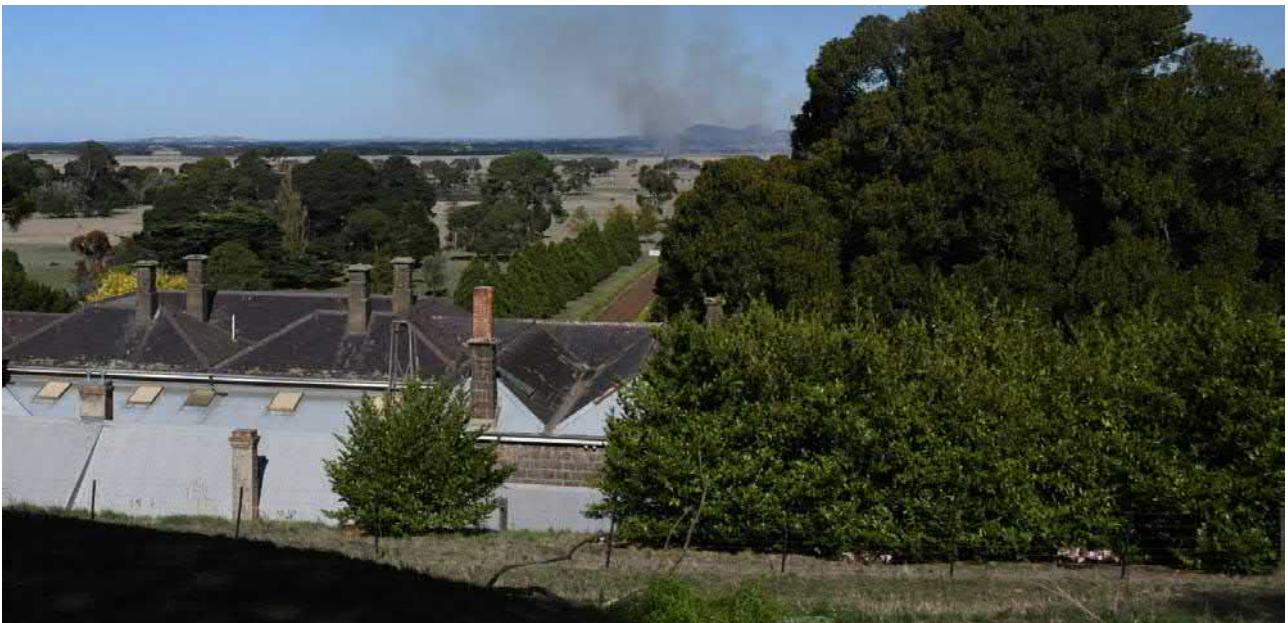
Figure 6-21: Viewpoint 10 – View over the top of the homestead
