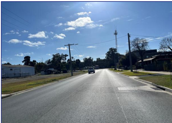
Figure 5: Sturt Street – view north
