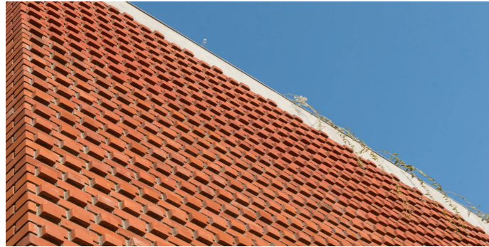
External Wall- East Elevation • Extruded Brick Texture
