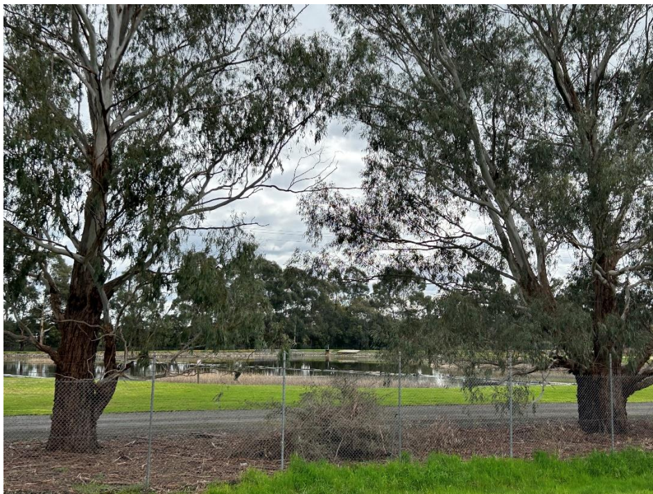
Photo C - The treatment plant ponds as viewed from the Yarra Valley Rail Trail
