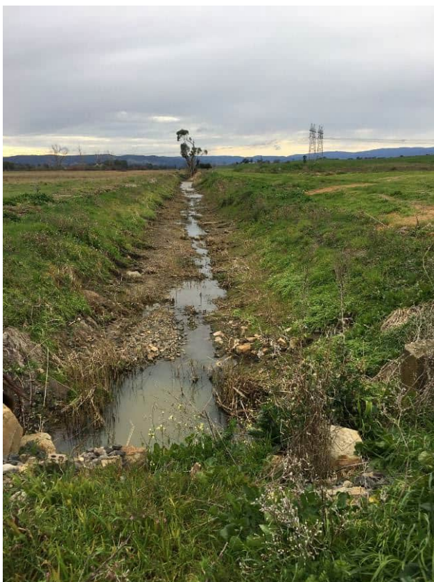
Figure 3.2: Nelson Road Drain clearing in 2017 previously cleared of native vegetation.
