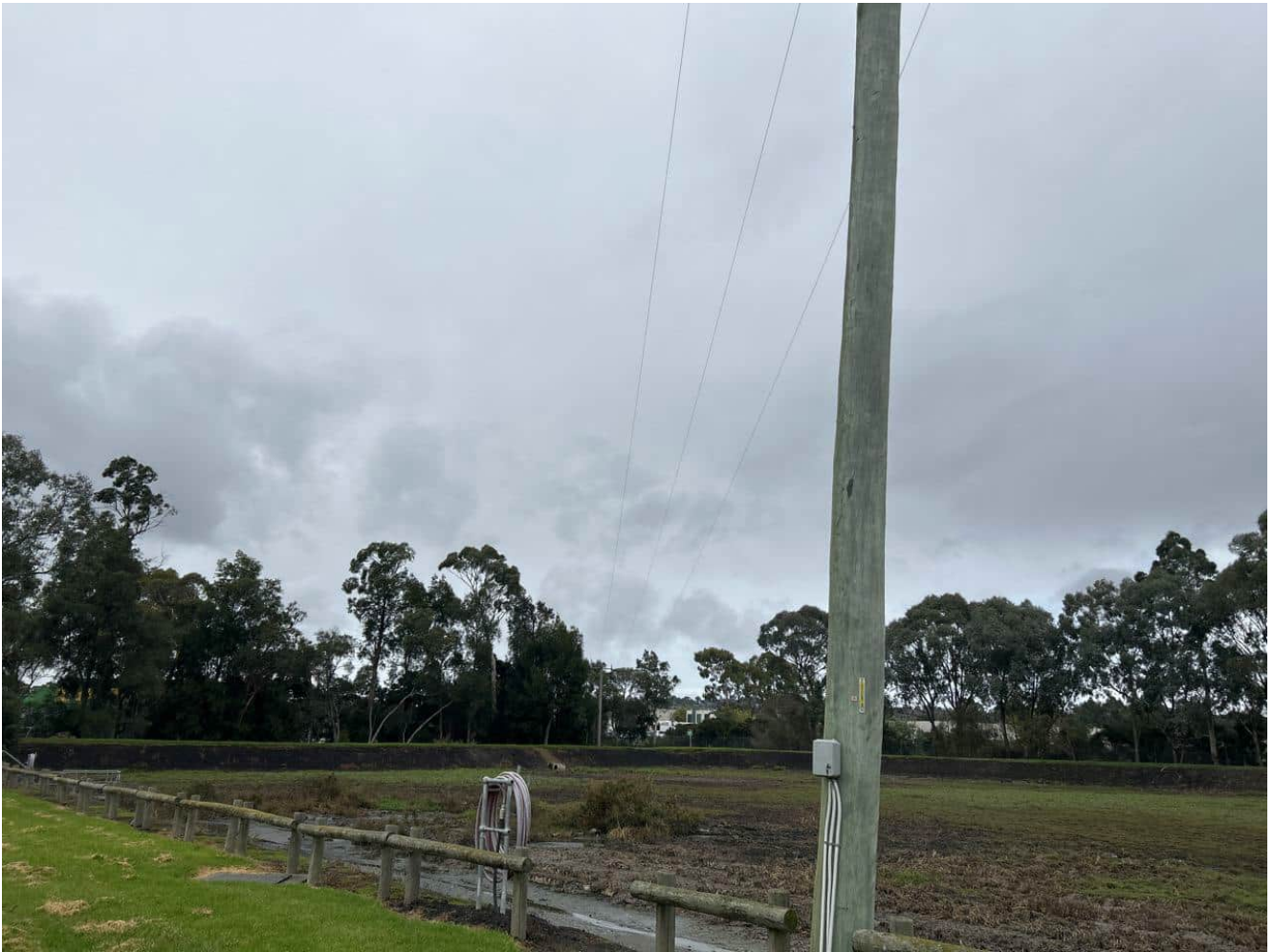
Figure 3.14: Artificial DEWLP mapped wetland: Lilydale Sewage Farm (South) (ID 71749) where the proposed powerline will be strung.
