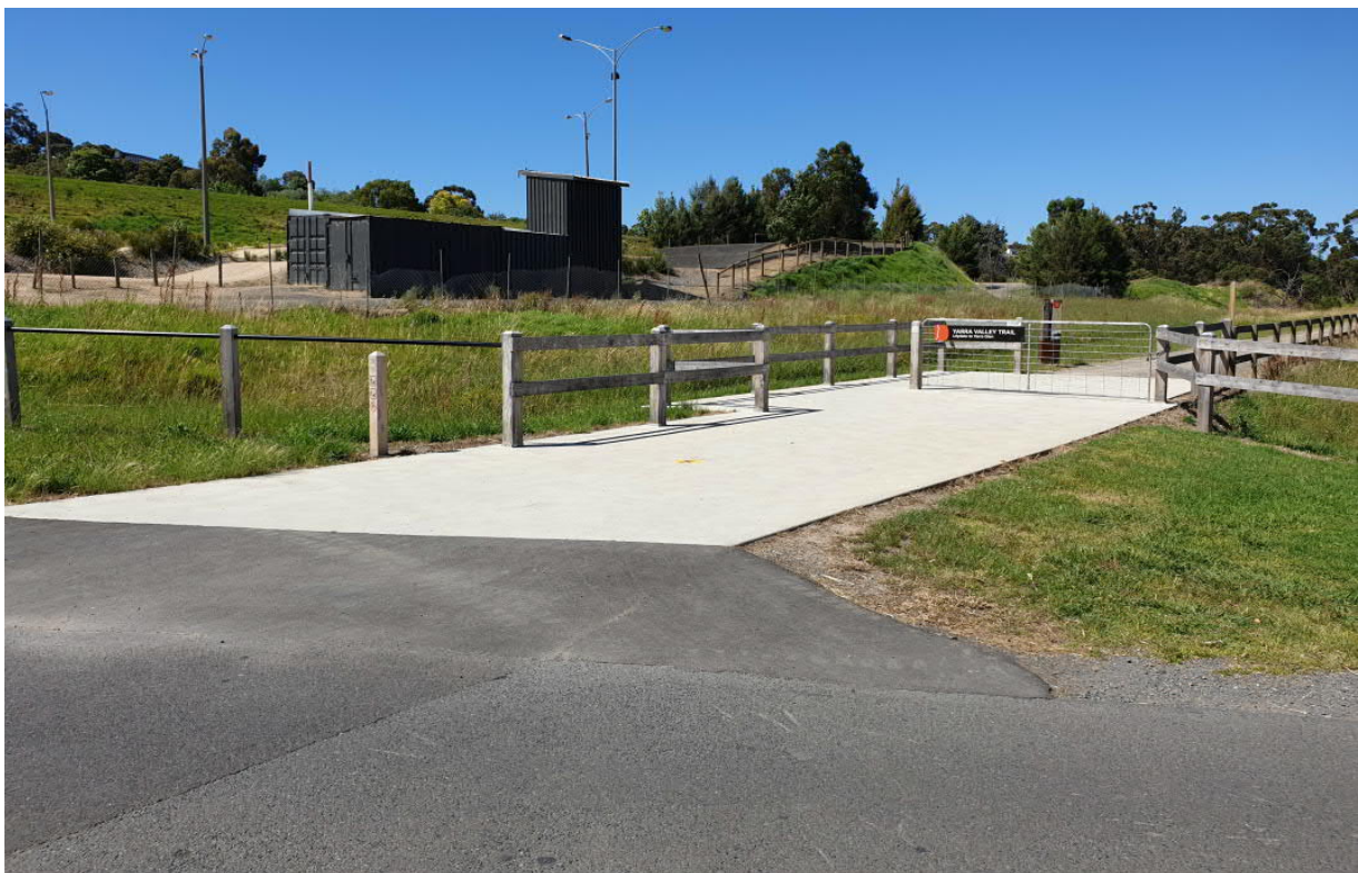
Figure 4: Access Road Typical Rail Trail Entry-Exit Treatment (Source: Yarra Ranges Council)
