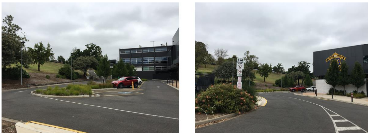
Figure 6-1 - Photo 1 – Car park to be removed and Library to the right of the photo
