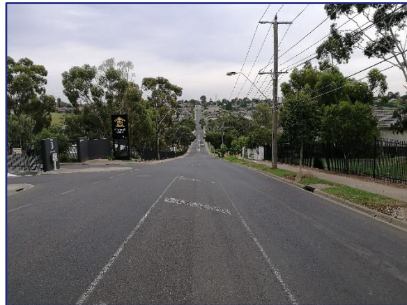
Figure 5: Rosehill Road - View West
