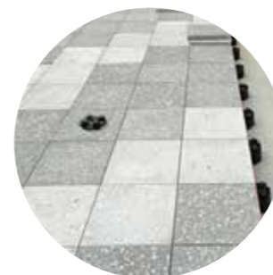
Pavers on a pedestal system
