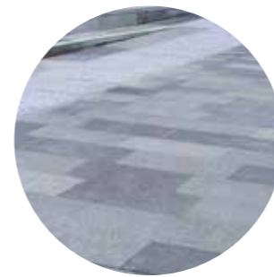
Unit paving to communal areas
