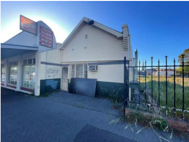
Figure 2: Front of existing building facing Barnard Street.
