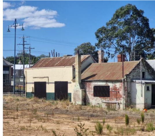
Figure 11: West (side) façade of 253 Barnard Street. The rear portion of the building appears to be an earlier structure compared to the front. Source: Trethowan Architecture, 2025.
