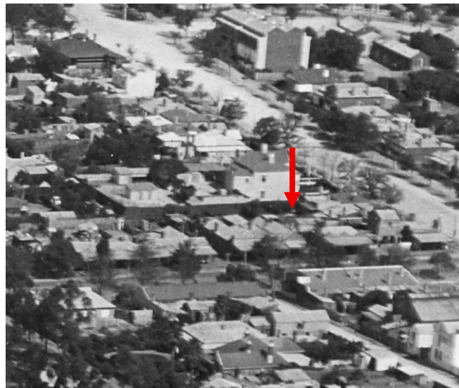
Figure 17: Section from a 1929 photograph, showing the western end of Barnard Street. Building at 253 Barnard Street indicated red arrow. Source: State Library of Victoria, Aispy photography collection.
