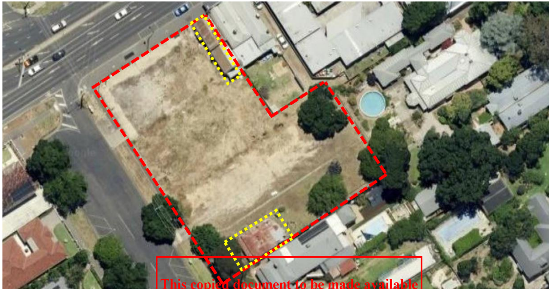
Figure 1: Aerial view of the site (indicated in red) with two extant buildings (in yellow). Source: Google Maps.
