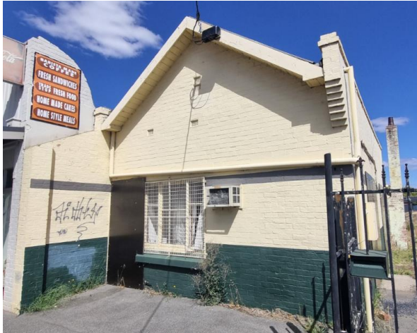
Figure 10: North (front) façade of 253 Barnard Street. Source: Trethowan Architecture, 2025.
