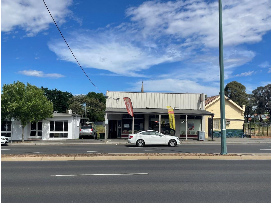
Photograph 7: No. 247-249 Barnard Street
