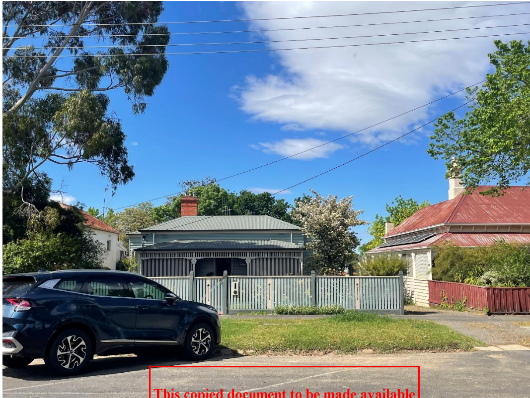
Photograph 8: No. 142 Wattle Street
