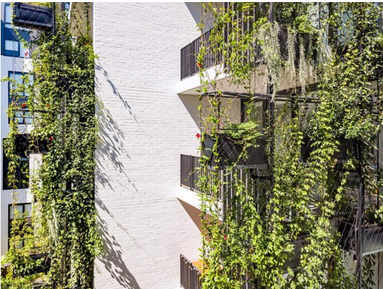
CONTINGENCY SOLUTION IN EVENT OF PLANTING FAILURE. STAINLESS STEEL WOVEN WIRE, THREADED THROUGH MESH. HEIGHT TO ALIGN WITH HEAD OF ADJACENT DOOR (2.4M NOM. FOR BALCONIES, 2.1M NOM. FOR MAISONETTE)
