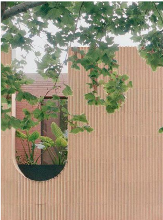
CN-1 RAKED PIGMENTED CONCRETE PROFILE: RECKLI 2/150 B-VOSGES OR SIMILAR FORMLINER PROFILE. MAX DEPTH 16MM. COLOUR: ABILOX CHAMPAGNE OR SIMILAR
