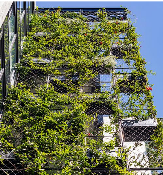
STAINLESS STEEL MESH AND PLANTERS PROVIDING SCREENING TO END OF BALCONIES AT VANCE APARTMENTS, HAROLD PARK, SYDNEY.
