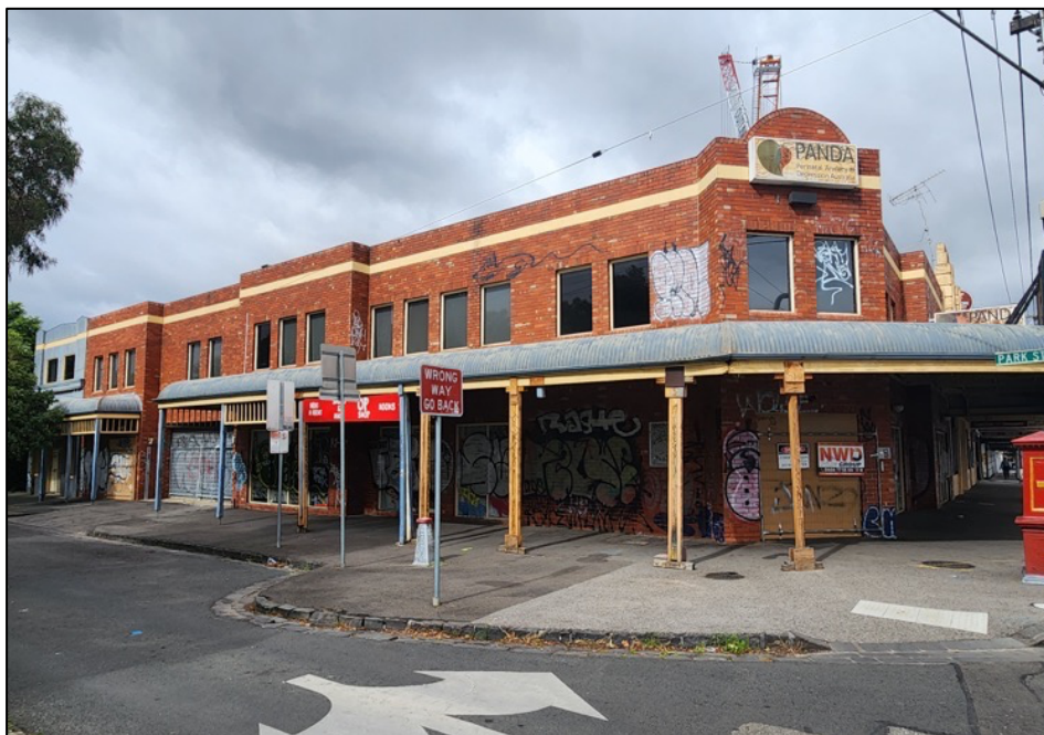
Figure 6 North elevation of the c.1970-80 building known as 806-810 Nicholson Street.
