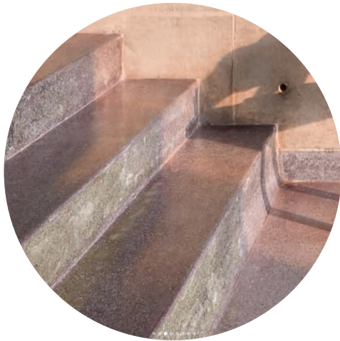
CN-3: Pigmented Concrete to match architectural specification
