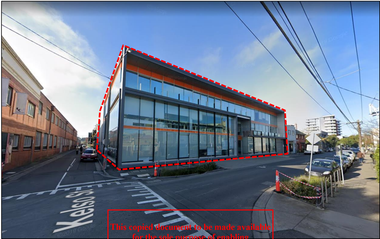
Figure 2 – Subject Site – existing under developed condition. (December, 2019).
