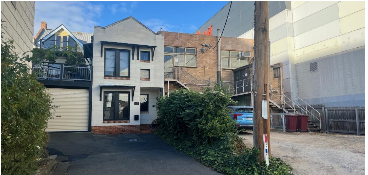
Figure 6: View towards 10 Hays Place and the rear of 159-161 Malop Street to the south of the site.
