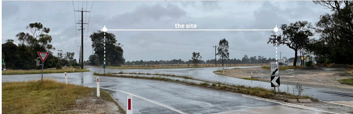
View to the site.
