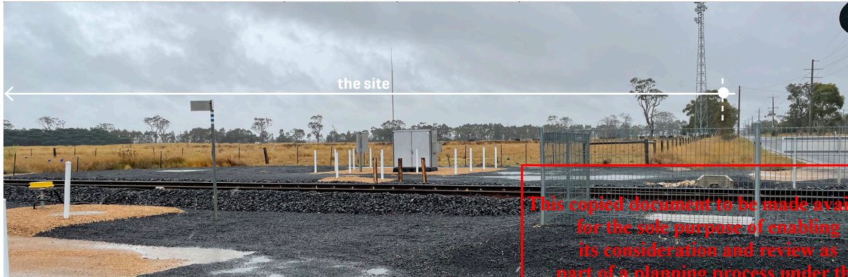
View to the site.
