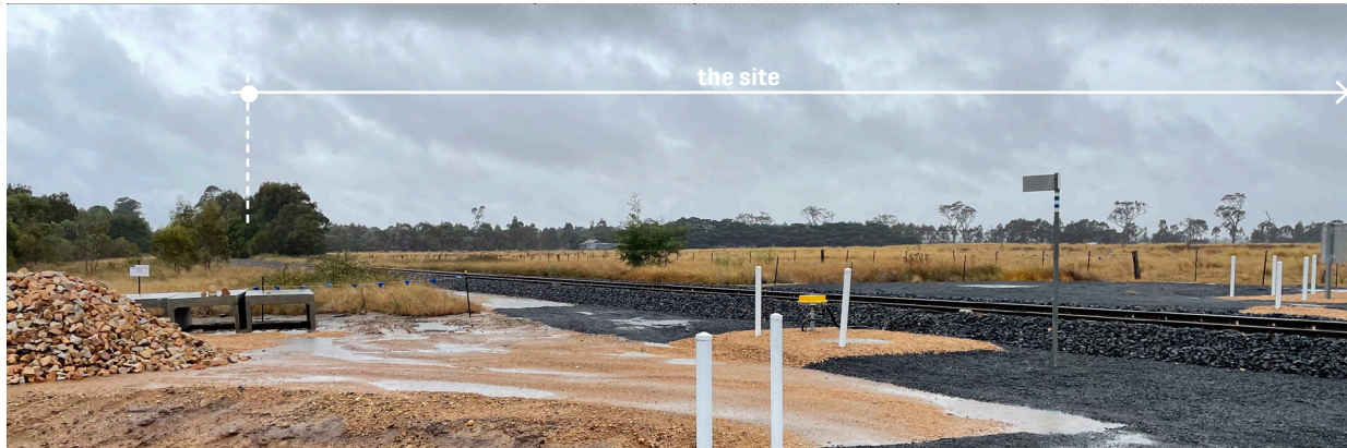
View to the site.
