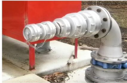
Figure 2: 125mm, 100mm, 90mm, 75mm, and 65mm Storz tree adapters.
