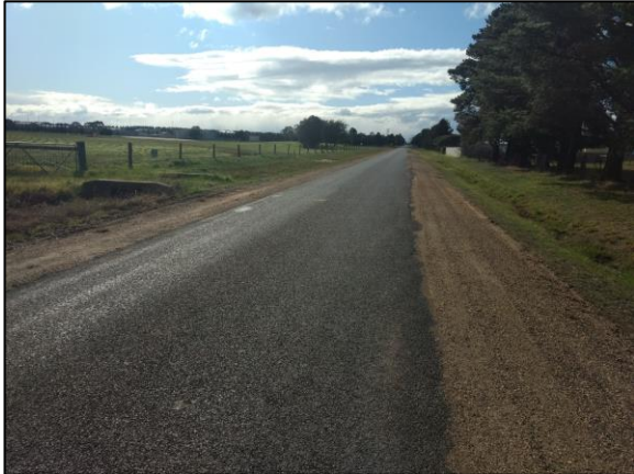
Figure 5: Hopkins Road - View North
