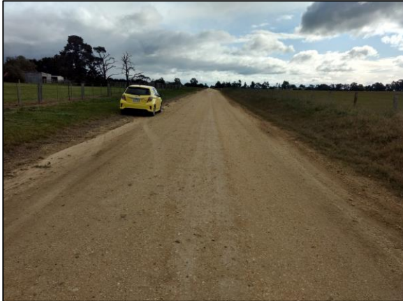
Figure 7: McLarens Road - View West
