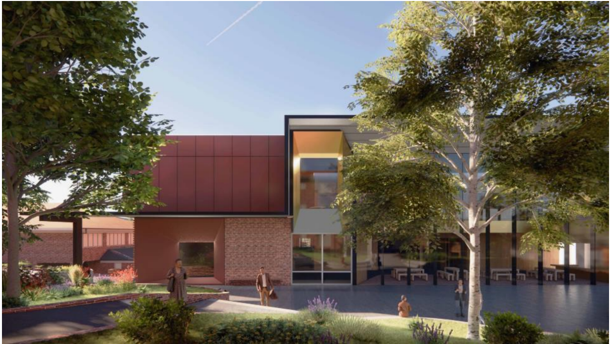
Figure 12: View internal to the school
