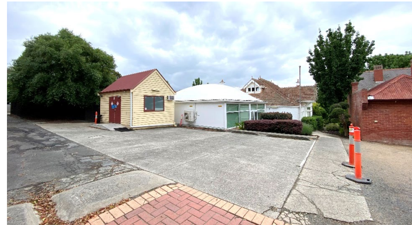
Picture 3 – Rear of parcels 2\PS332542 and part of 25\LP4997
