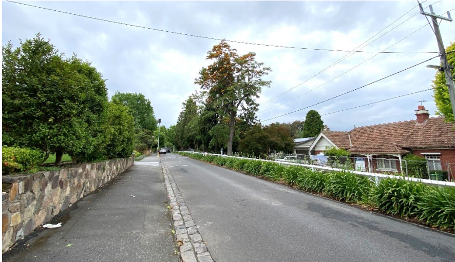
Figure 4 – Marshall Street, adjacent to the site
