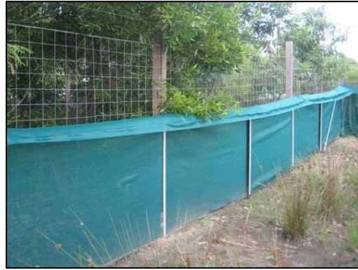
Plate 2: Temporary fence for amphibians, made of silt fencing (Source: Jake Urlus, Tactecol)
