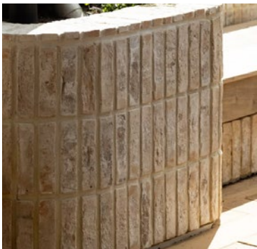
Brick planters & terraces
