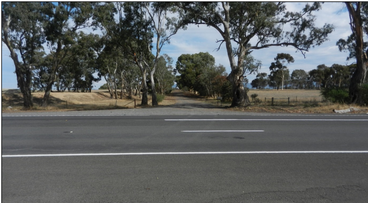
Photo 5 - The existing farm driveway to No. 4785 looking south across the Western Highway.
