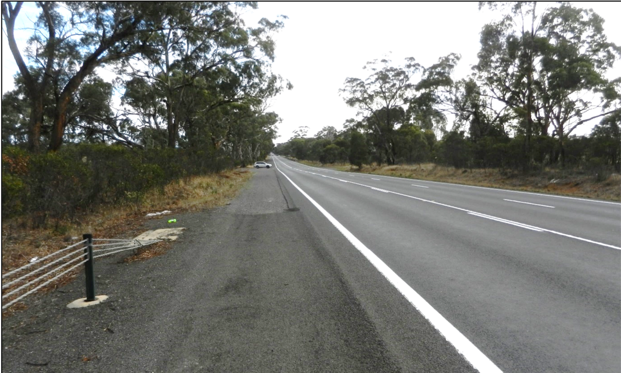
Photo 4 – View to the southeast showing gap in shoulder sealing downstream from the property entrance.
