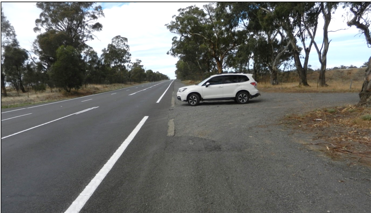
Photo 4 – View to the southeast showing gap in shoulder sealing downstream from the property entrance.
