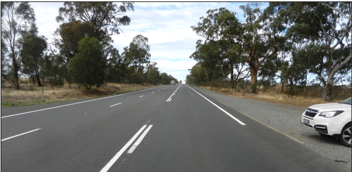
Photo 1: View to the southeast at the subject property driveway showing lane configuration of Western Highway.
