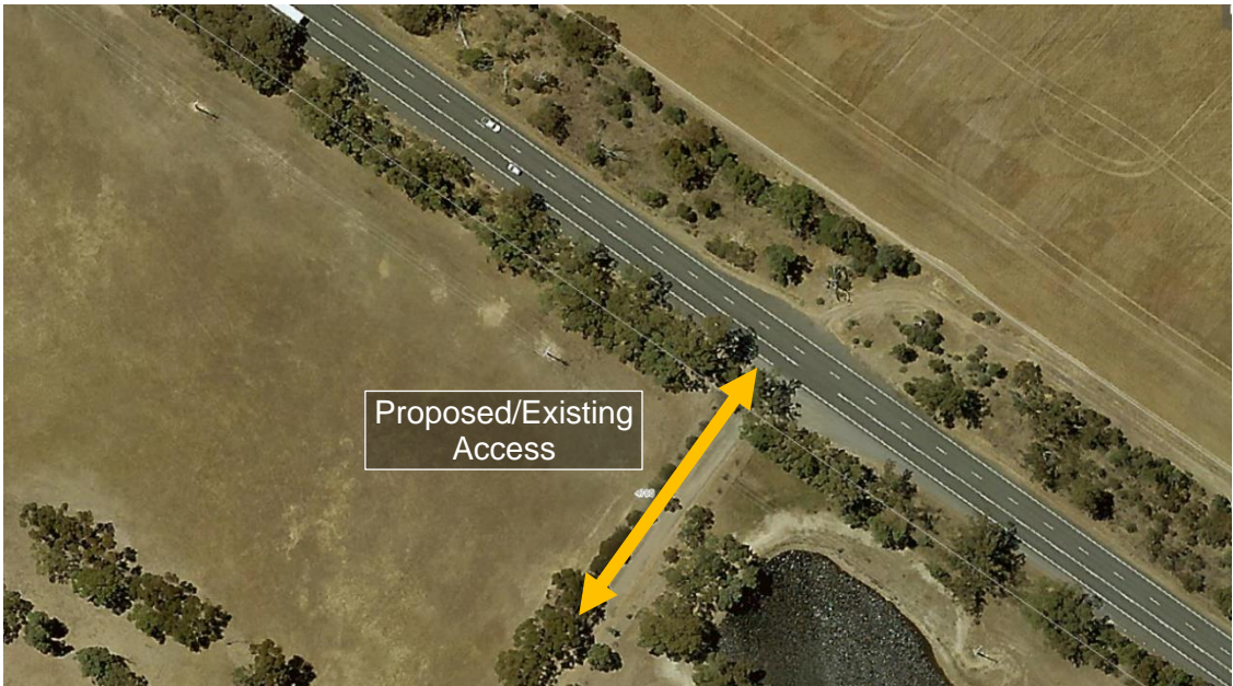
Figure 15. Existing Road Conditions – 4785 Western Highway
