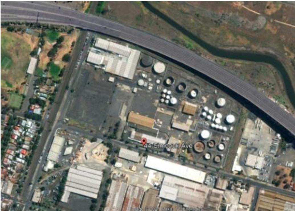
Figure 3 - Site Layout Prior to Demolition (2013)
