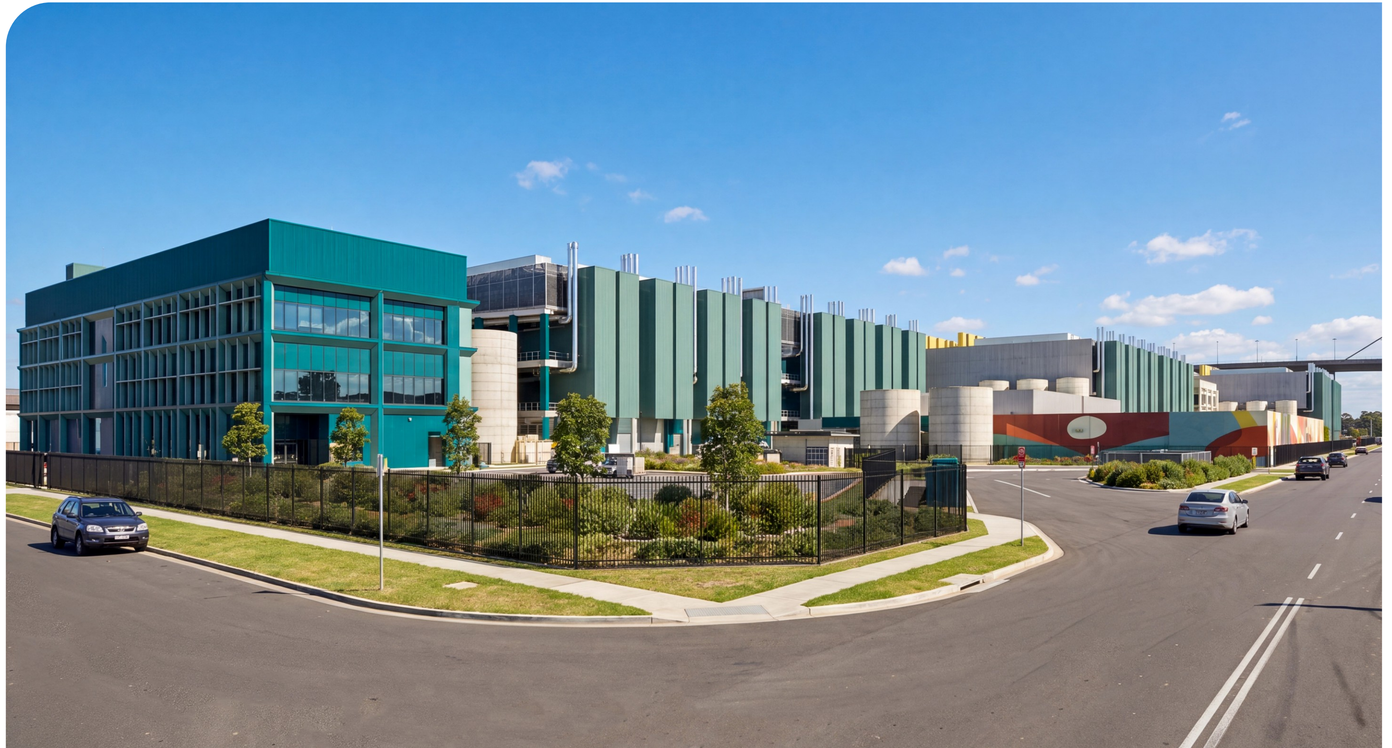
View from Hall street - Simcock Avenue
