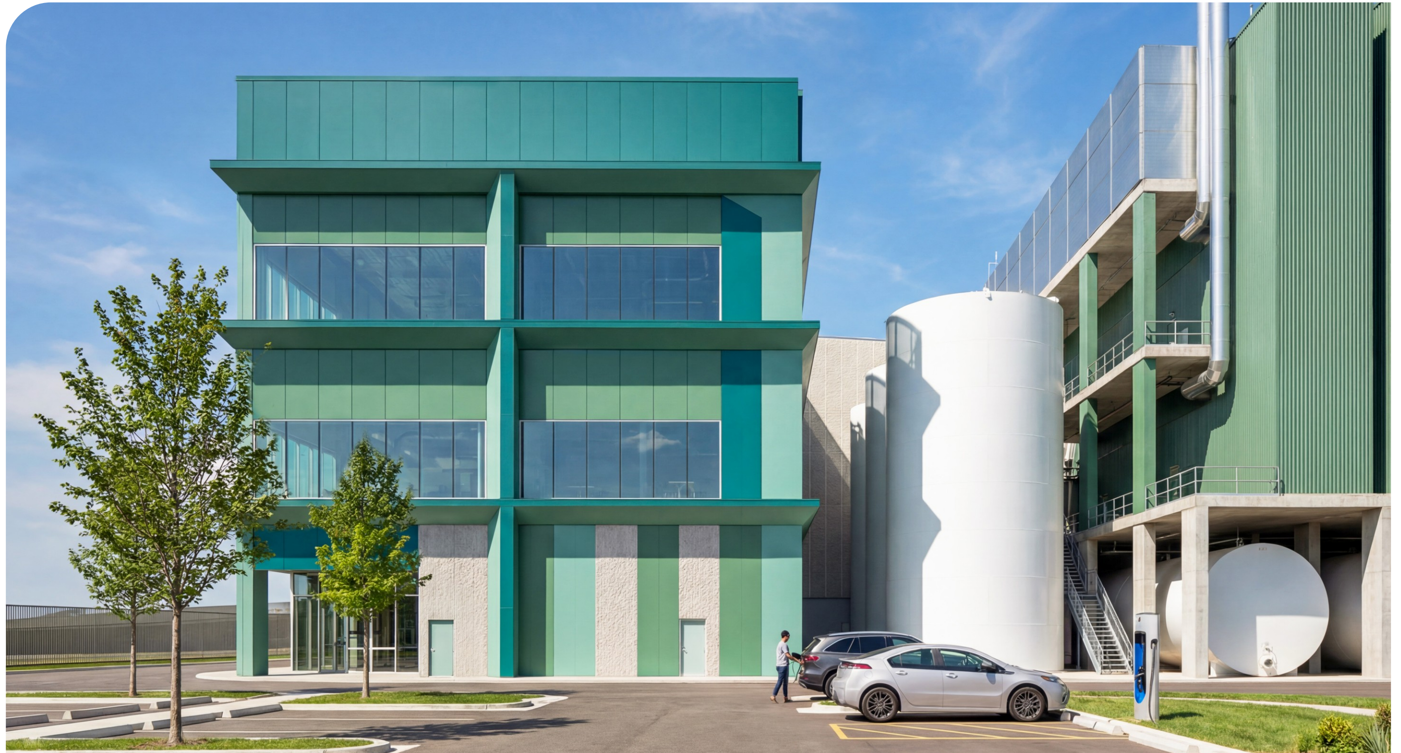
Tech Building B View
