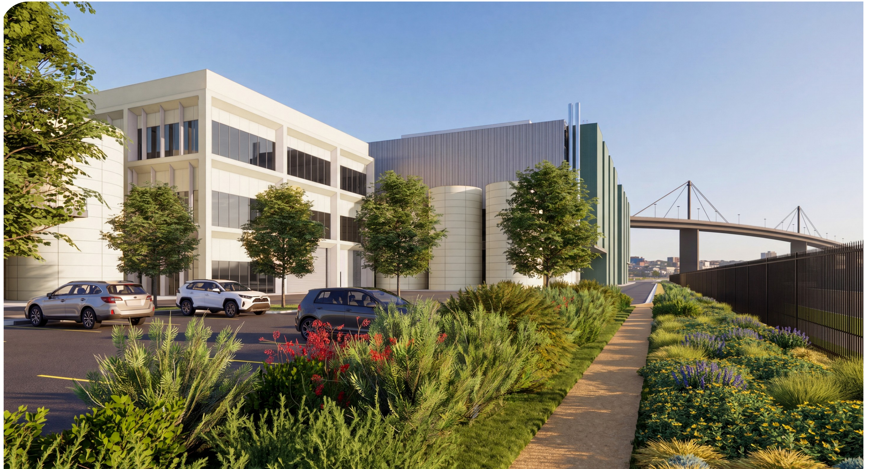
Tech Building B View
