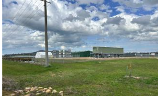
Figure 8: view of site from intersection of Chivers Road/Winton-Glenrowan West Road
