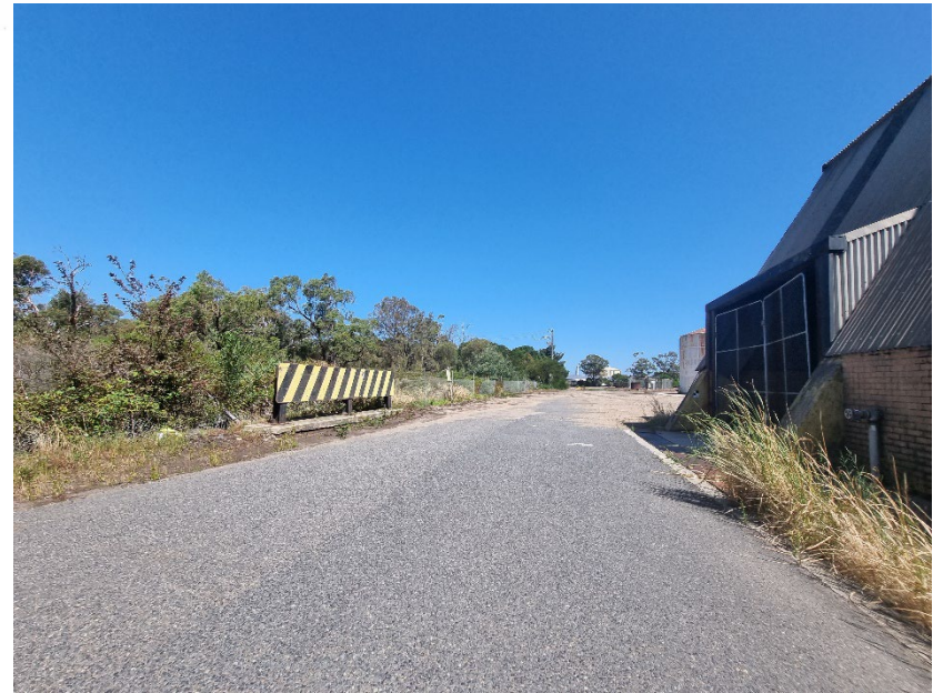
19. View looking south, along the eastern elevation of warehouse.
