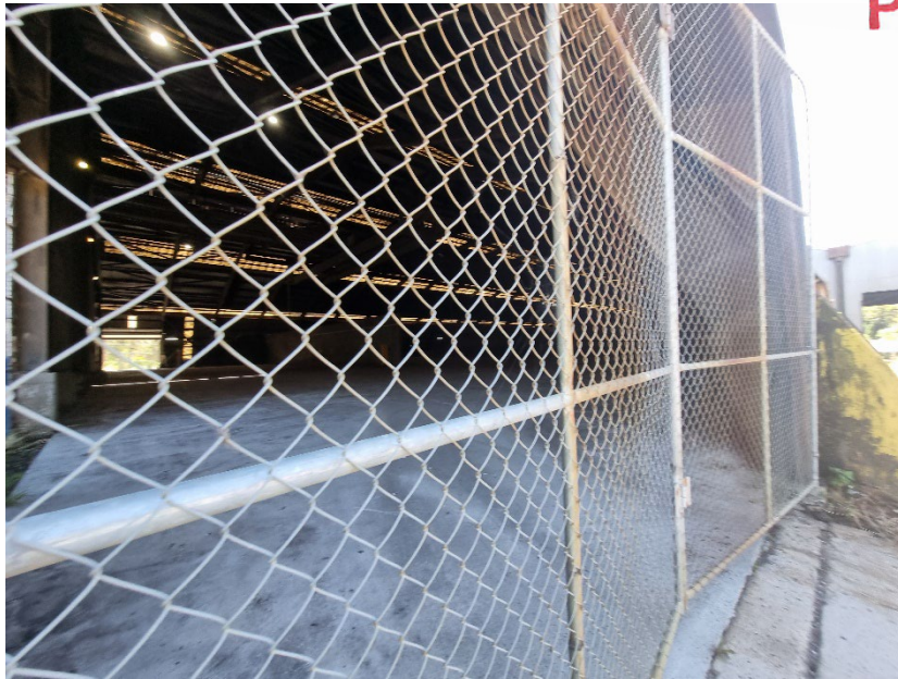
17. View into the (vacant) warehouse building.
