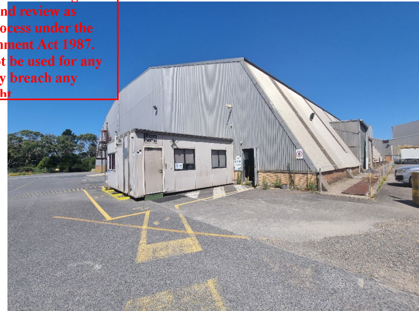
3. Front of existing building (warehouse) to Lot 40 (north elevation).
