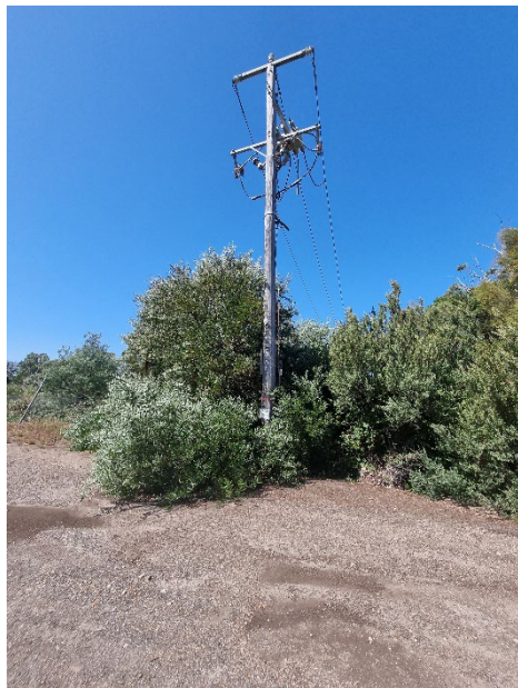
14. Existing power Lines located to the eastern boundary of Lot 39.
