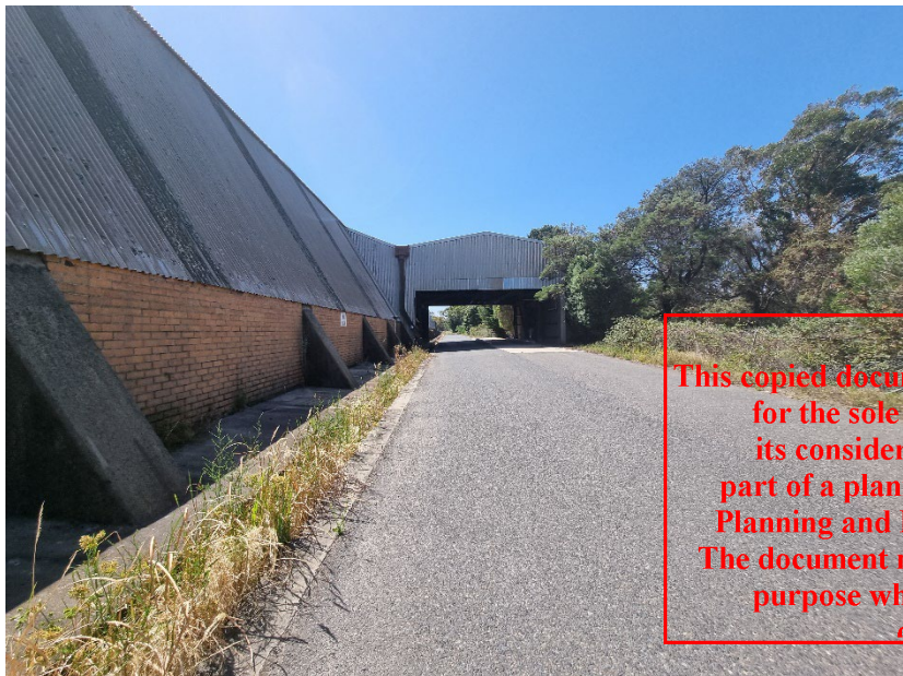
18. Looking north, along the eastern elevation of the warehouse.
