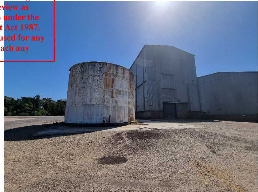
15. View to existing building and water tank to Lot 40.
