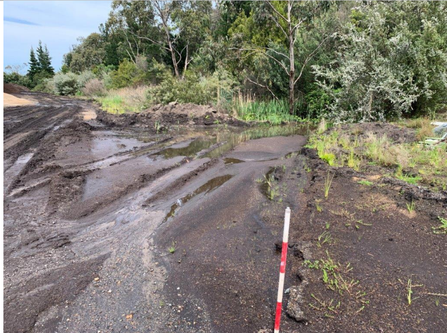
Plate 3: View of pooling water along the western edge of the gravel pad (Matthew Barker 8/10/21) facing southwest
